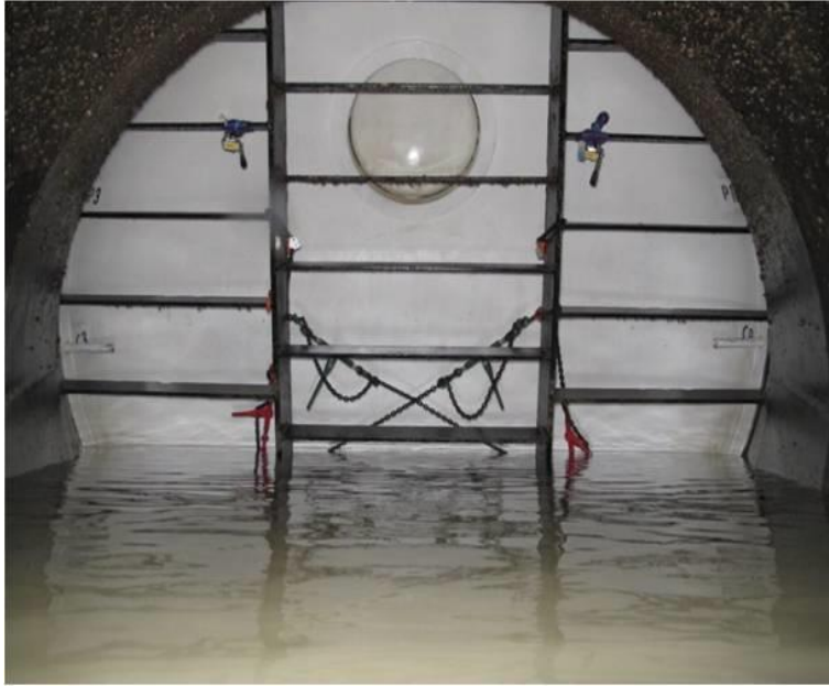
Fig. 4. View from downstream face of a bulkhead, during dewatering of outlet
