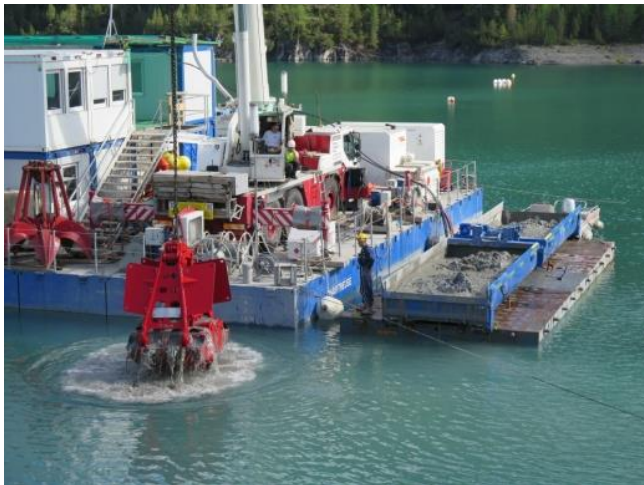
Fig. 2. Grabbing operation at -110 meters
